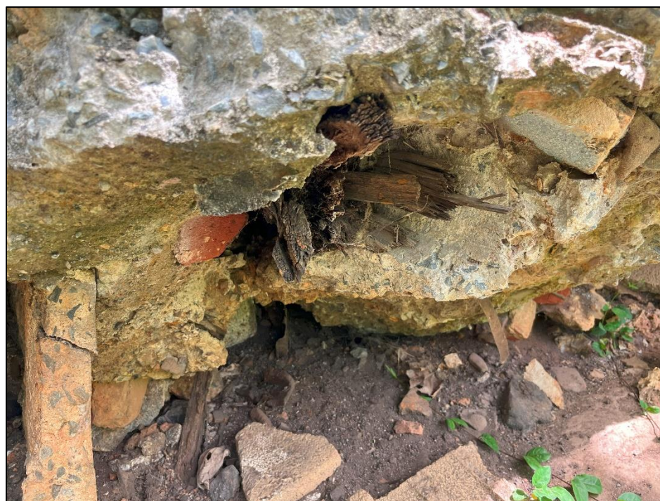
Figure 46. Photo showing handmade bricks and potential remains of a wooden crib dam or sluice encased in concrete on left bank of Ivy Creek. Photo by J. Gantzert.
