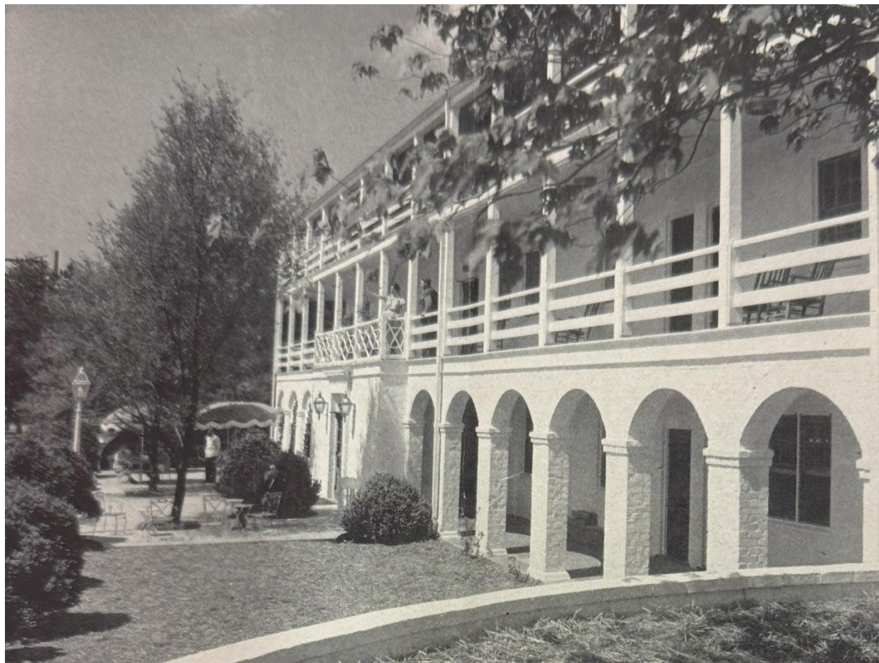
Figure 14: As described in The Hotel Monthly , published in July 1951: “The south wing showing covered porches, from which entrance is made to guest rooms. This view shows the dining terrace and the transient entrance to the dining room. There is also an entrance to an interior stairway leading to the galleries off which guest rooms are located. For isolation of noise and easy access to playground areas, the four guest rooms behind the arcade are intended for guests traveling with children. There is an extensive parking area to the left of the picture.” ( The Hotel Monthly , Milton L. Grigg Papers, Albert and Shirley Small Special Collection Library, University of Virginia)
