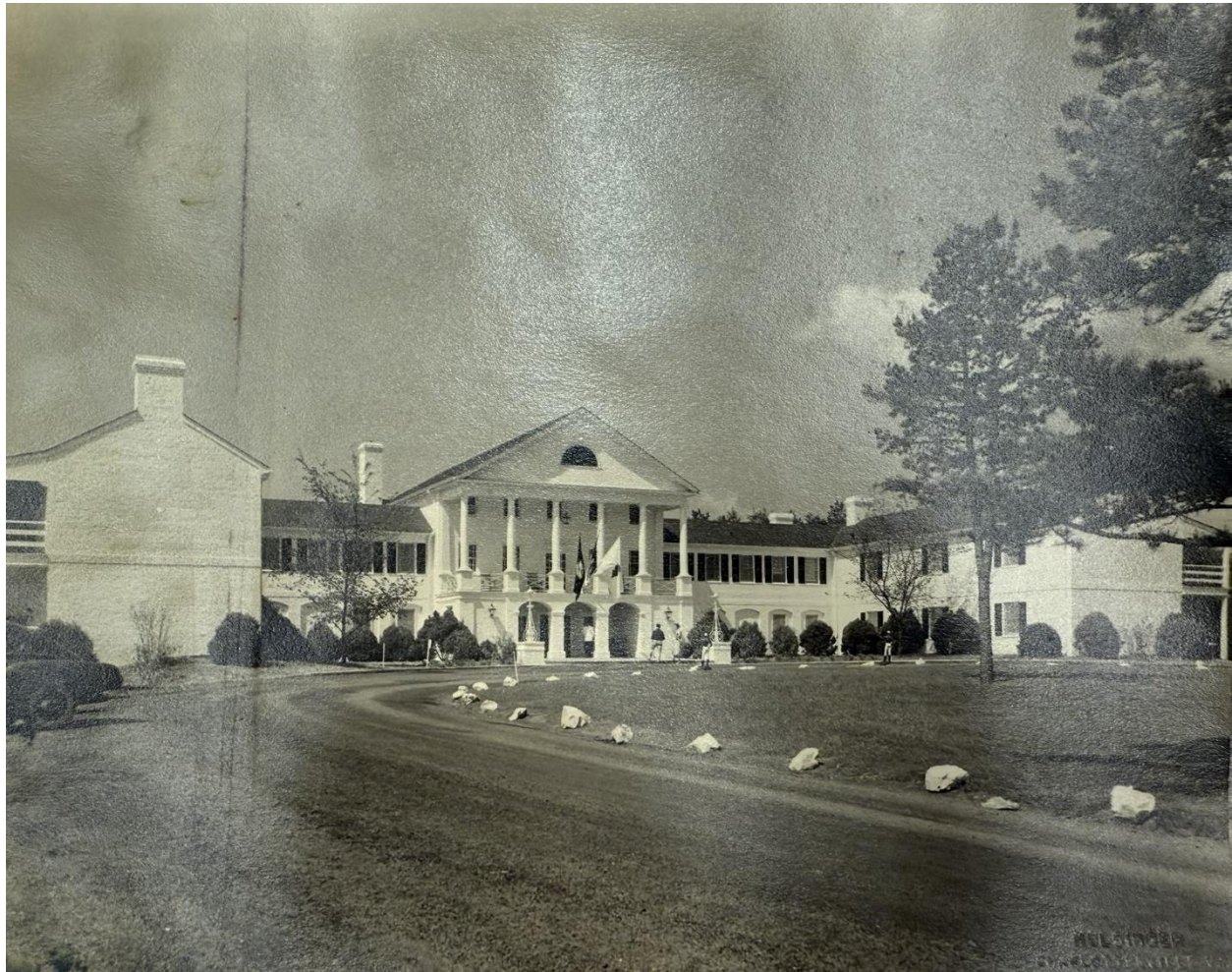
Figure 12: Completed Thomas Jefferson Inn looking west, c. 1951. (Milton L. Grigg Papers, Albert and Shirley Small Special Collection Library, University of Virginia)
