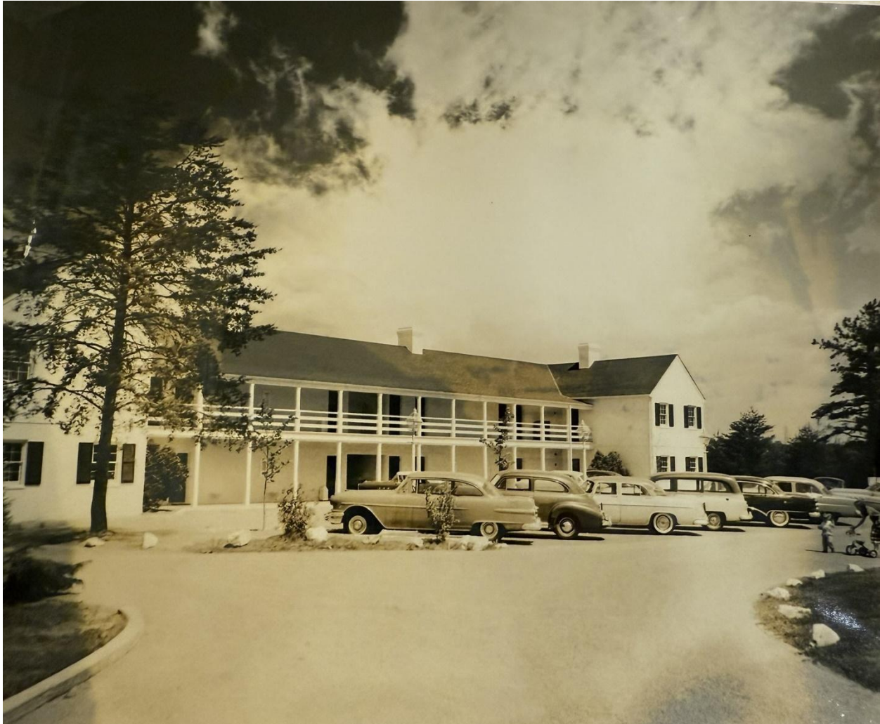
Figure 19: Completed Annex Building, c. 1956. (Milton L. Grigg Papers, Albert and Shirley Small Special Collection Library, University of Virginia)
