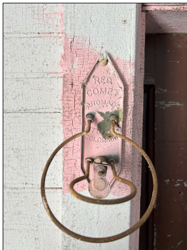
Figure 6. Bracket for historic-period fire extinguisher in the north section of Rocky Branch School (Image Source: Commonwealth Preservation Group, 2025).
