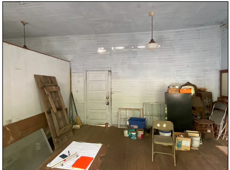
Figure 3. At left, framing beneath exterior siding indicates former door location; at right, beadboard wall covering indicates former door opening (Image Source: Joseph D. Lahendro, historic architect, 2025).
