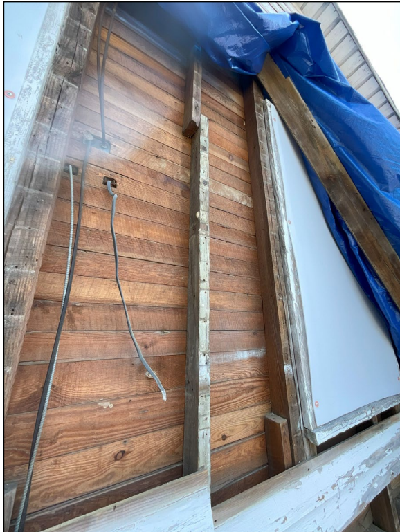
Figure 3. At left, framing beneath exterior siding indicates former door location; at right, beadboard wall covering indicates former door opening (Image Source: Joseph D. Lahendro, historic architect, 2025).
