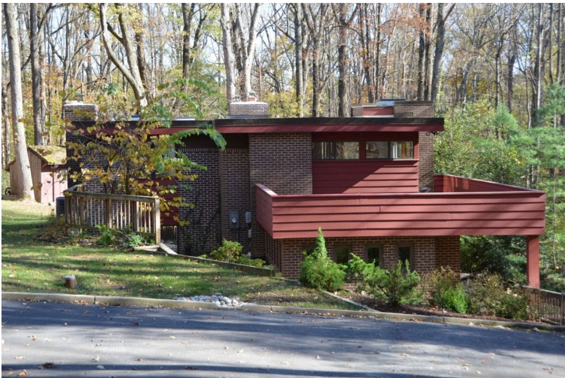
Figure 24. Rollo Residence (DHR# 029-6592), Fairfax County, 2019. Photograph, VCRIS.
