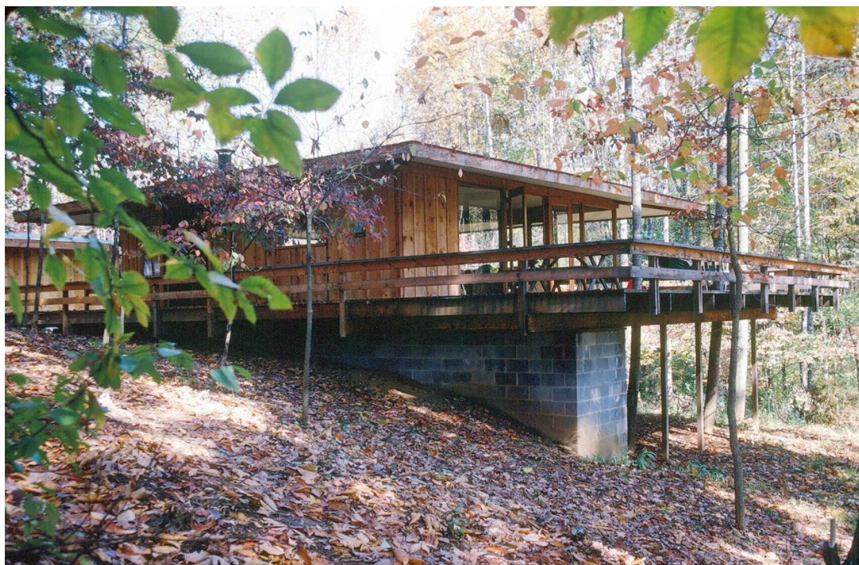
Figure 23. The Holden Residence, c. 1964, 8600 Chandler Street, Fairfax VA. Photo undated, NCModernist Chandler .
