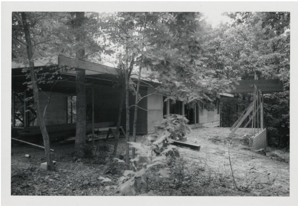
Figure 13. The Hammond House under construction, ca. 1962.
