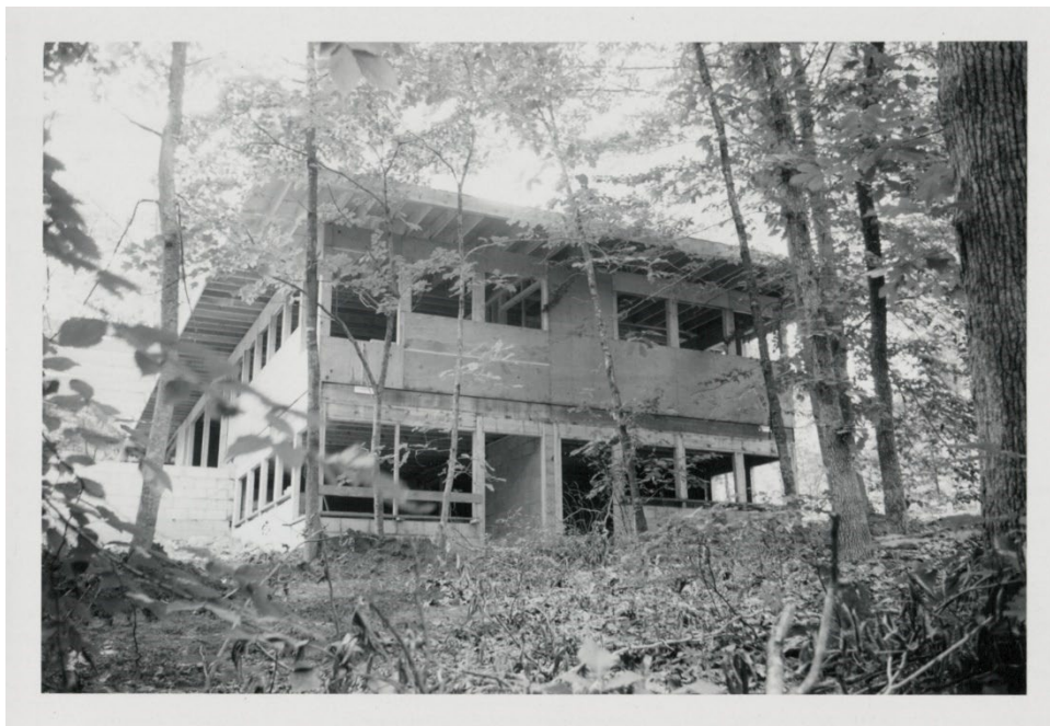
Figure 14. The Hammond House under construction, ca. 1962.
