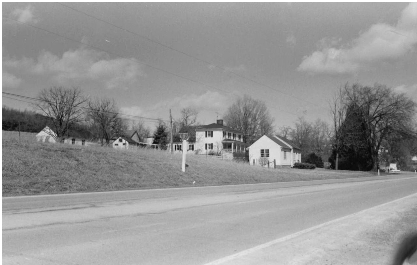
Figure 4. Mint Spring Tavern, photograph from April 1973 Virginia Historic Landmarks Commission survey. (Virginia Department of Historic Resources)
