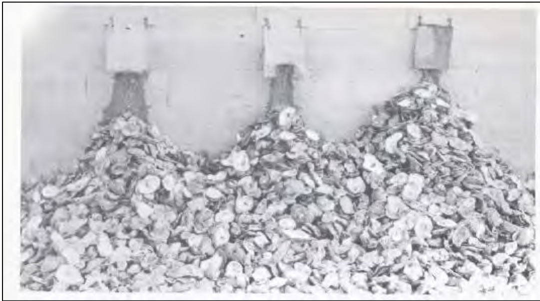
Figure 11: Oyster holes on the exterior of a typical shucking house. These holes on the exterior of the concrete block structure had a functional purpose for disposing of and collecting shells, and now make oyster houses from the period an identifiable resource. This shucking house may have been referred to as a “three-hole.” Ca. 1990. From Close Ties: Reflections from Rappahannock Watermen.
