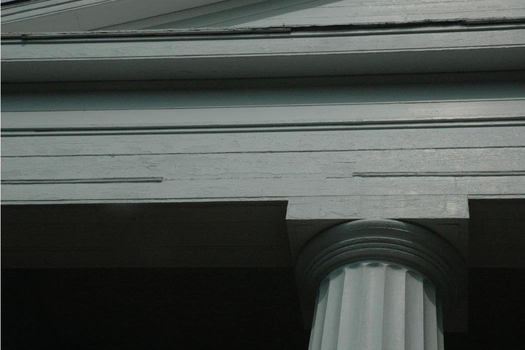
*Figure 19. Missing section of molding on architrave of portico.*
