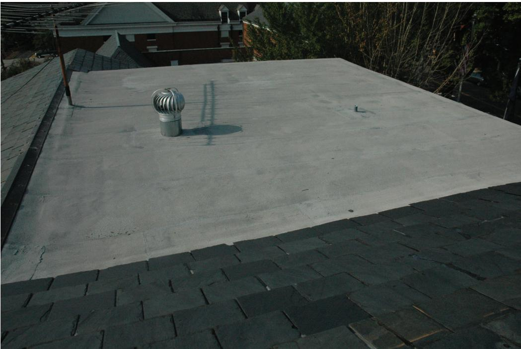
*Figure 15. Asphalt roofing on flat deck.*
