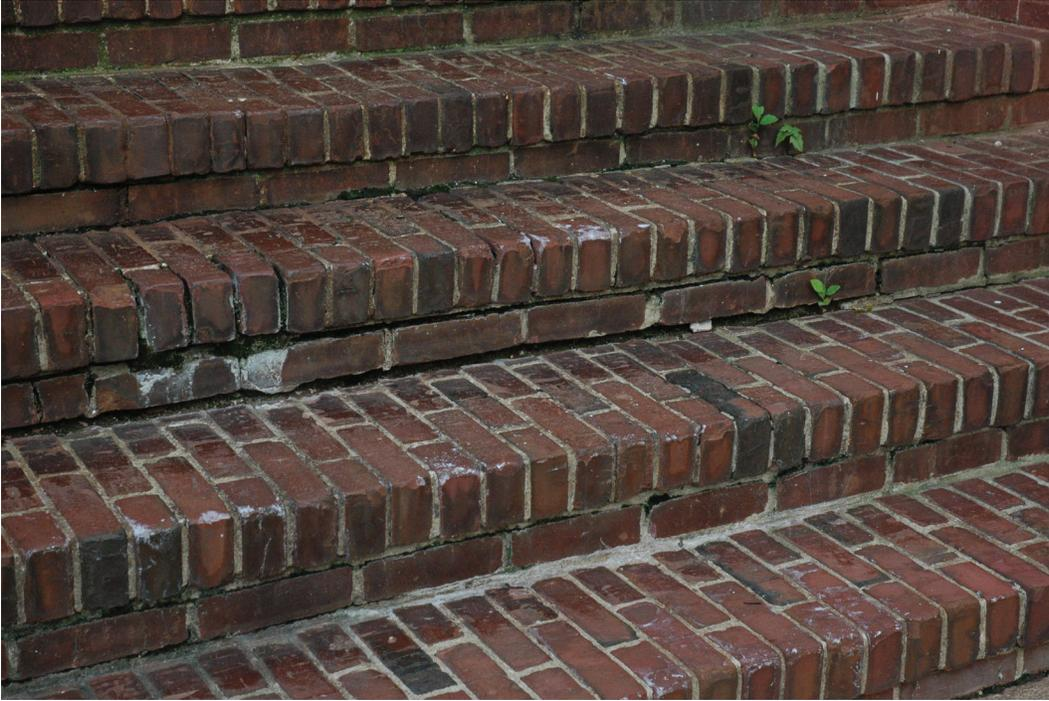
*Figure 29. Failed mortar joints of north porch – 1939 wing.*
