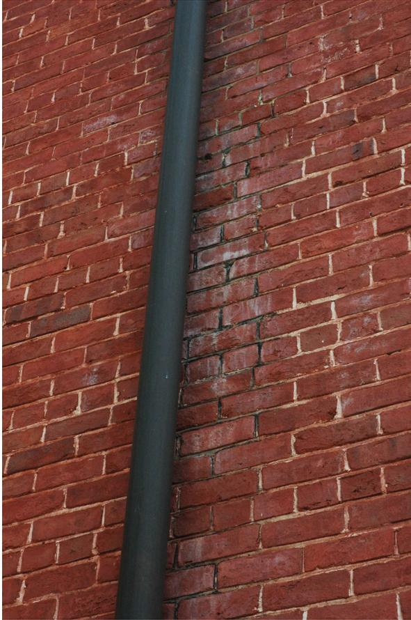
Figure 26. Wall stained by blocked rain leader.
