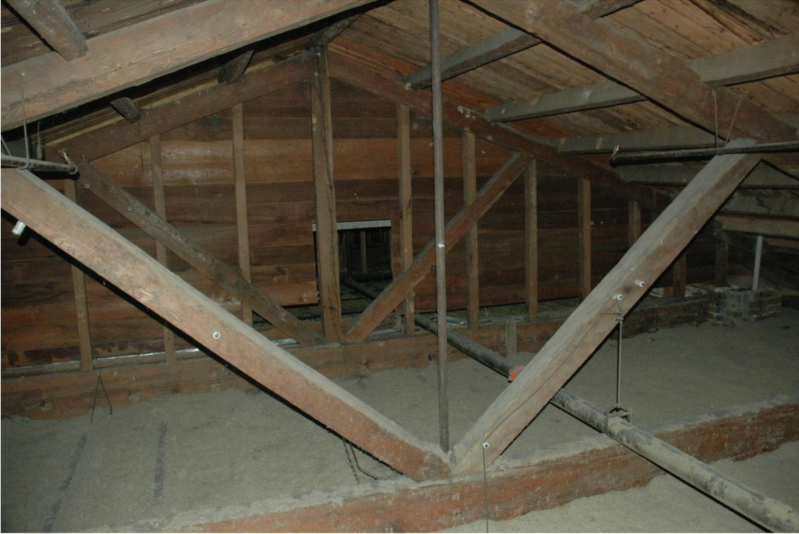
*Figure 47. Trusses in 1854 attic.*
