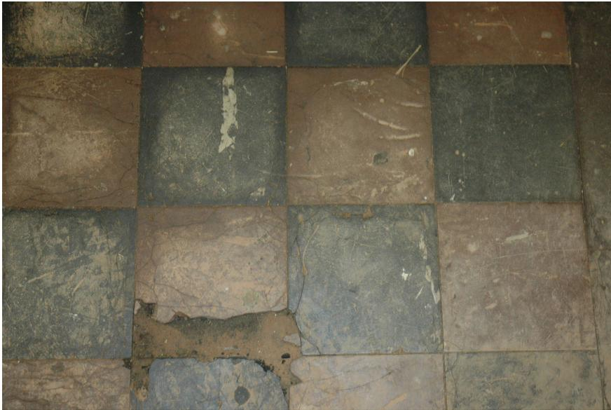
*Figure 62. Destroyed floor tiles in Room B8.*
