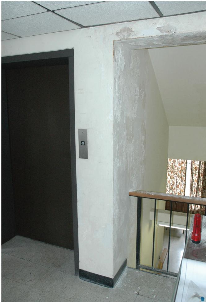
*Figure 56. Damaged plaster at the elevator shaft.*
