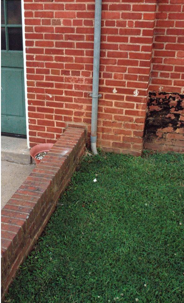
*Figure 39. 1939 waterproofing and ghost of higher cheek wall at north entry.*
