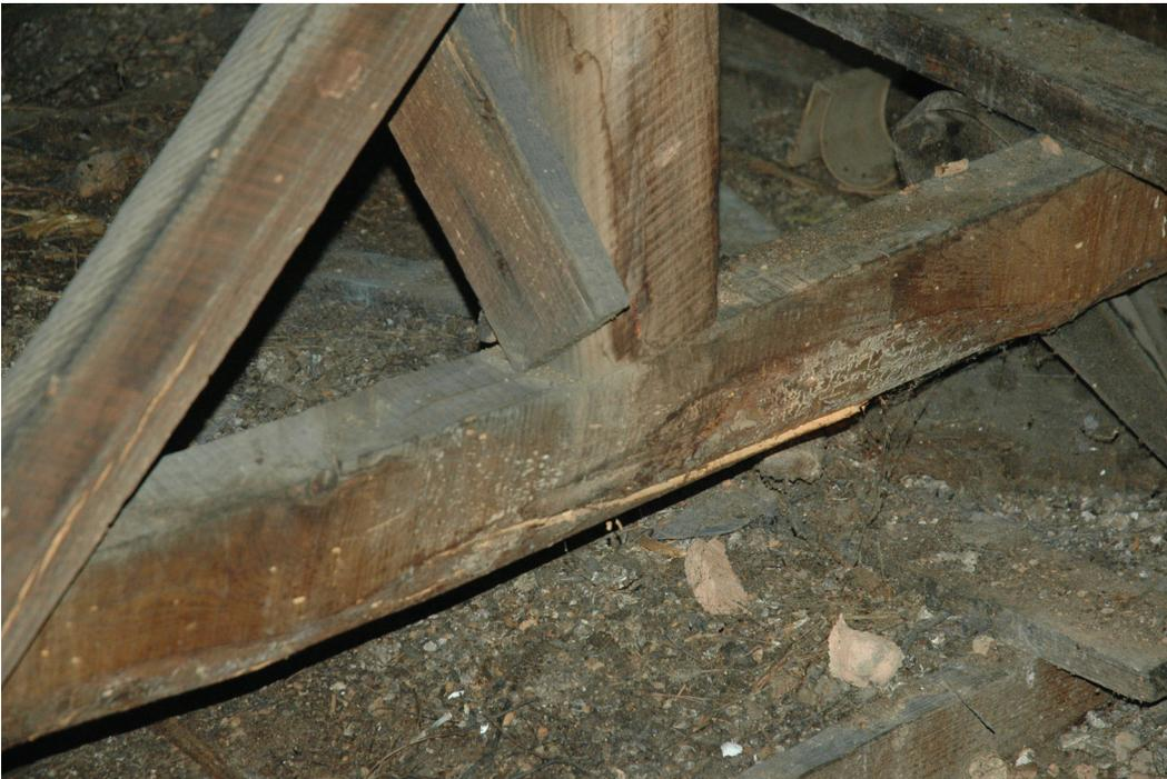
*Figure 48. Sagging girder below northeast corner of the cupola.*
