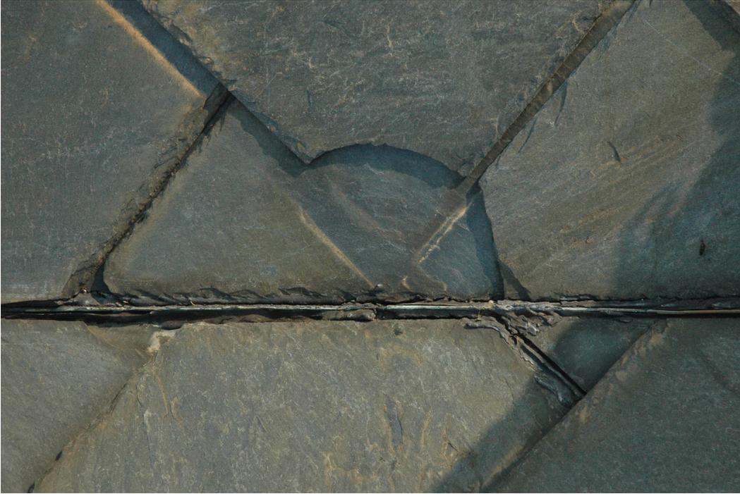
*Figure 14. Closed valley of slate roof.*
