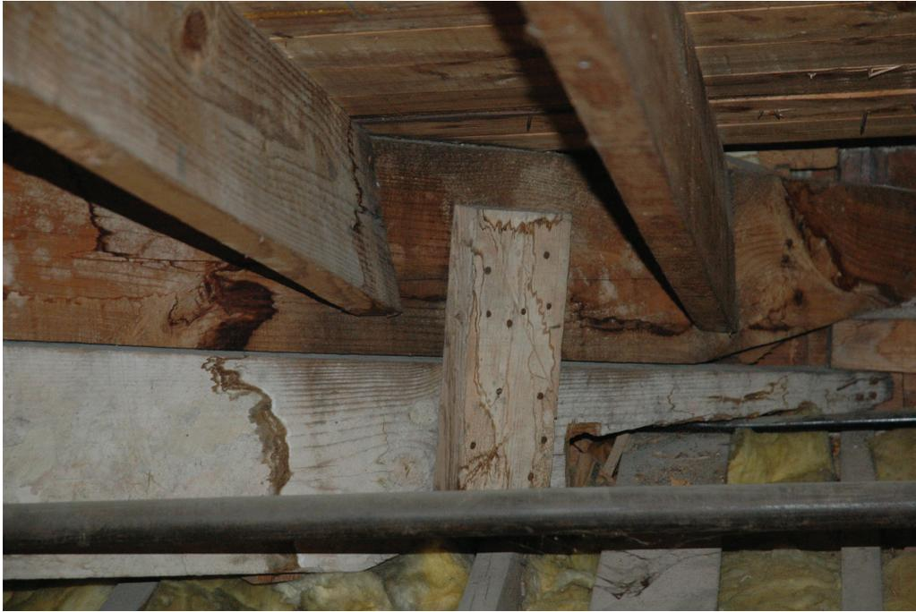
*Figure 52. Evidence of roof leak – 1939 attic.*
