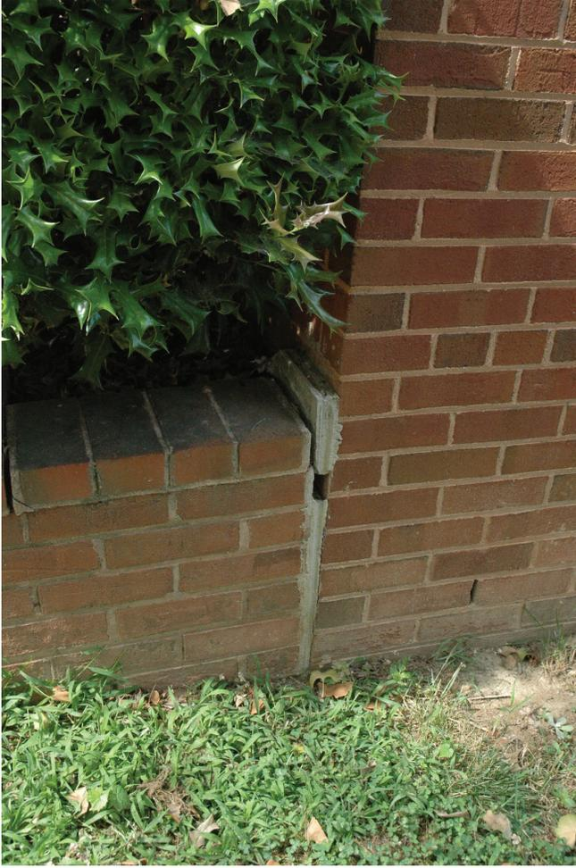
*Figure 44. Planter has rolled away from west face of 1976 addition.*
