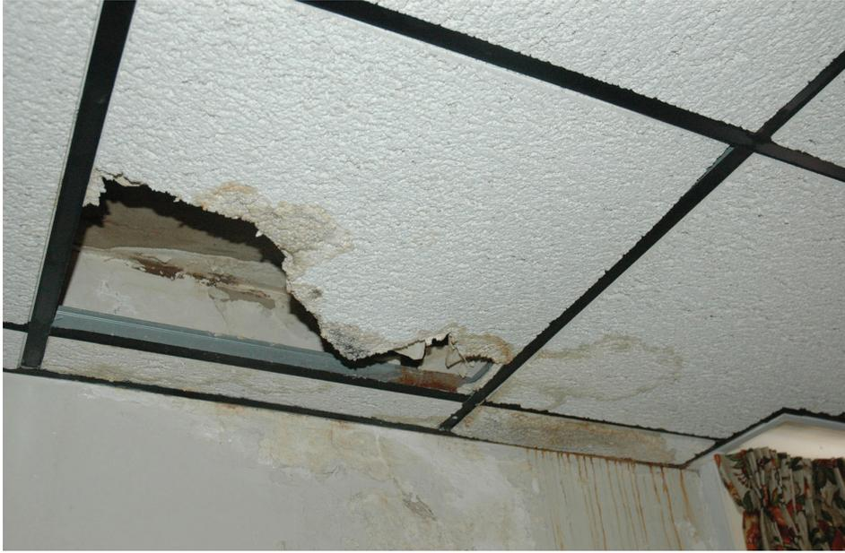
*Figure 55. Damaged ceiling tiles in Room 313.*
