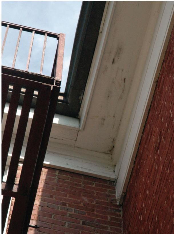
*Figure 22. Damaged cornice on the north façade of 1854 building.*
