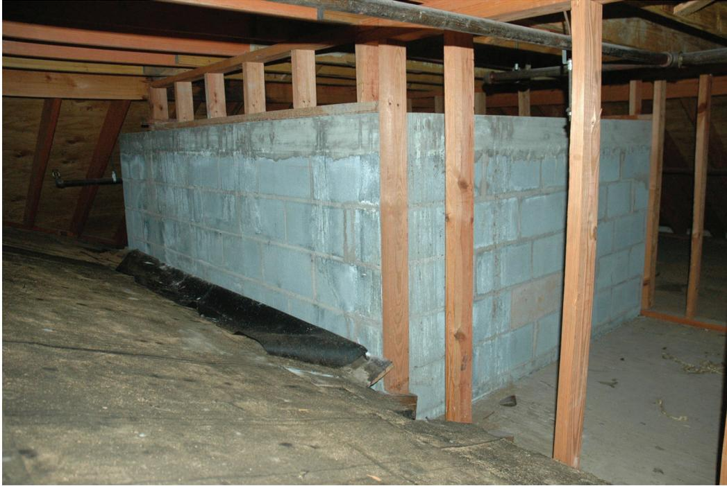
*Figure 54. Evidence of water running down sides of elevator shaft.*
