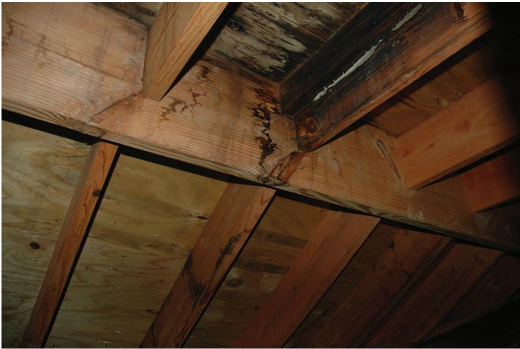
*Figure 53. Damage from leaking at eastern edge of flat roof deck.*
